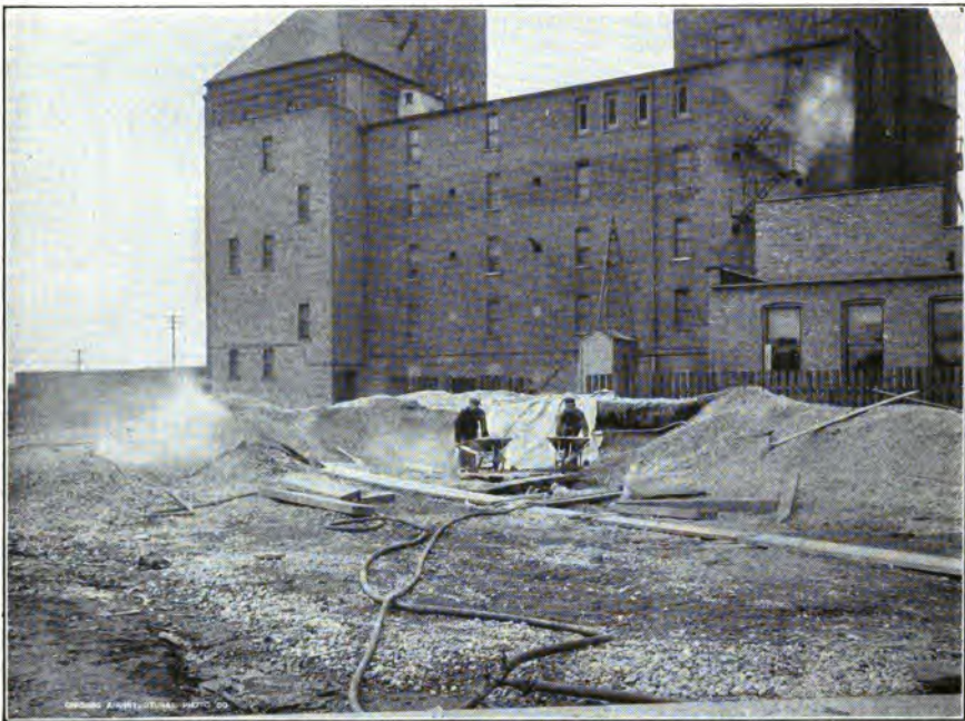
FIG. 3.—HEATING STONE PILE WITH STEAM. Canvas covering to retain all heat possible.
